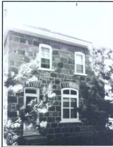
Killarney Baldwin Residence Built in the late 1890s, probably by the Hossack Brothers, figure 5, above. Similar stone working, asymmetric window and door placement. This building is gone. The survey page notes that the Hossack Brothers were noted for their ability to smooth out the rough surfaces of their stone faces. From: Survey of Killarney Manitoba . Manitoba Culture, Heritage and Tourism, Historic Resources Branch.
