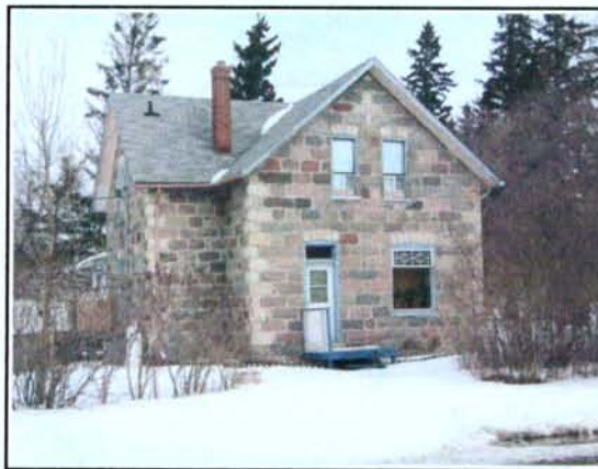
Sellar's House, built by Tom Bowyer in the late 1890s is still extant, figure 6 above. Note the course work, window headers and asymmetric placement of the openings. The same colorful choice of stone as Coghlan Castle, but a geologist has not examined this building to compare type of stone. The photograph is by Dale Bentley, February 2008.
