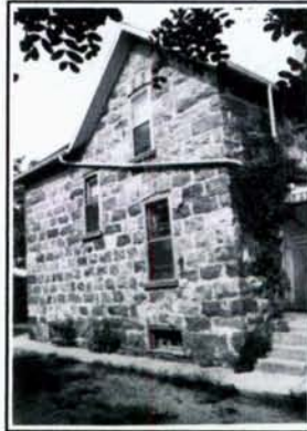
Thomas Bowyer's own residence, no longer extant. Built in the 1890s, figure 7 above. From: Survey of Killarney Manitoba . Manitoba Culture, Heritage and Tourism, Historic Resources Branch.
