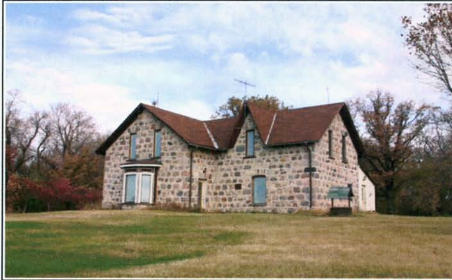
The McKenzie House 1892, Rapid City Area, built by stone mason T.D. Taylor, figure 9 above.
