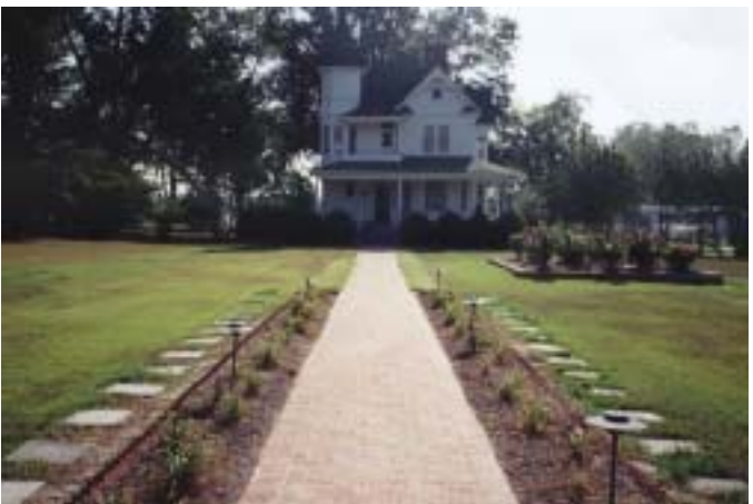
Historic Manager's Residence
