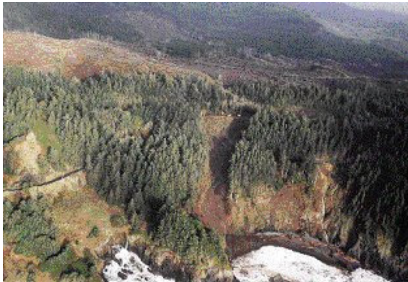
Figure 10. Cape Foulweather landslide. The downslope lanes of coastal US Highway 101 was damaged from a fill slope failure in December 1999. Repair work lasted about one month. (ODOT photo)
