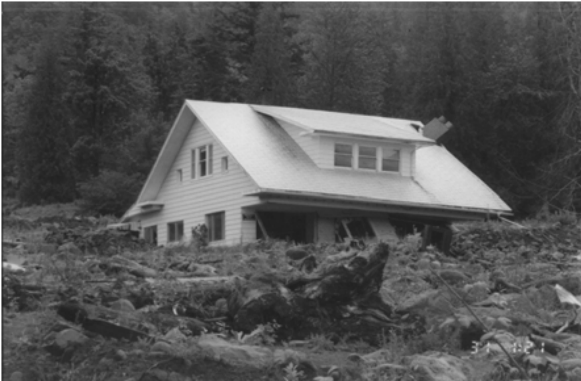
Figure 5. A debris flow destroyed this 2-story residence in Dodson, Oregon in the February 1996 FEMA-OR-1099-OR disaster.
