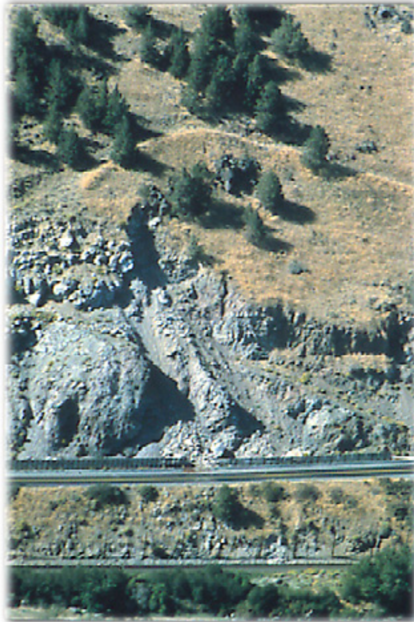
Figure 14. The 1993 Klamath Falls earthquake triggered a fatal rockfall on US I-97.
