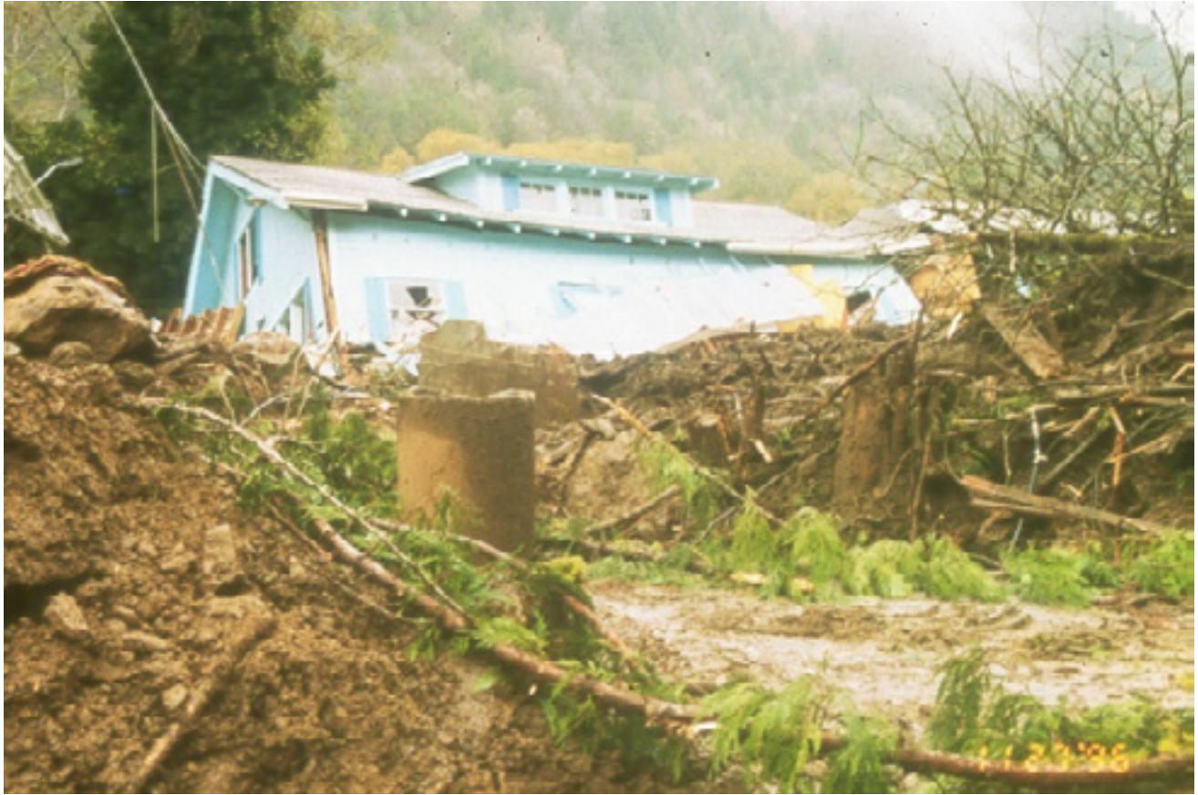
Figure 6. A debris flow destroyed this residence in Scottsburg, Oregon, in late 1996.
