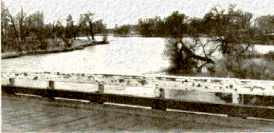
LOOKING UPSTREAM FROM EXISTING BRIDGE
