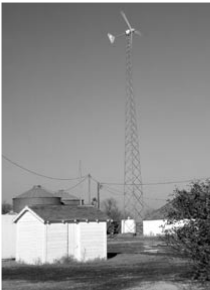
Warren Gretz, NREL/PTW09634
