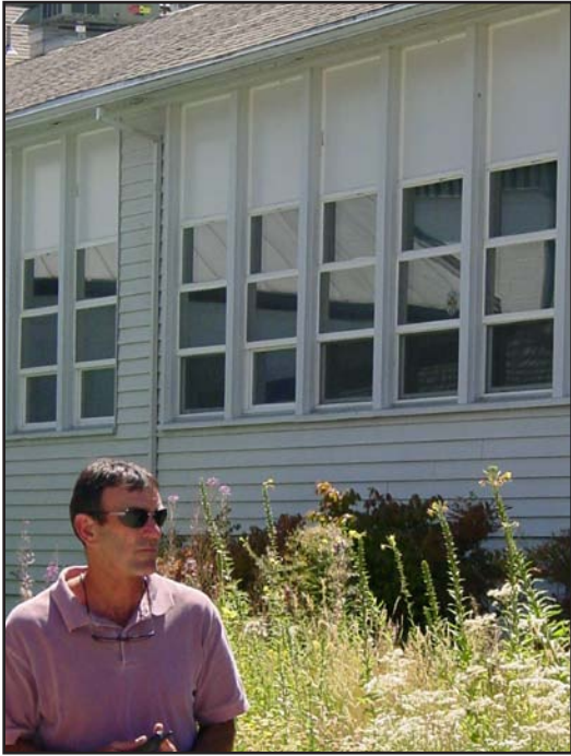
Tom Ries, facilities manager at Philomath School District, discusses his options in dealing with roof-top units.
