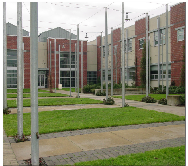
The Pine Street campus of Silverton High School incorporated daylighting measures on the windows to “bounce” more natural light into the classrooms. The poles were placed in the courtyard to serve as a trellis for vines to help reduce heat during hot sunny days. However, the plant selection was not appropriate and the vines never materialized.
