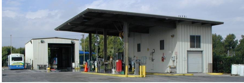
Figure C-2. CNG fueling lane and bus wash (Thousand Palms)
