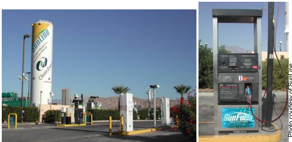
Figure C-1. Public fueling at SunLine's Thousand Palms CNG fueling station
