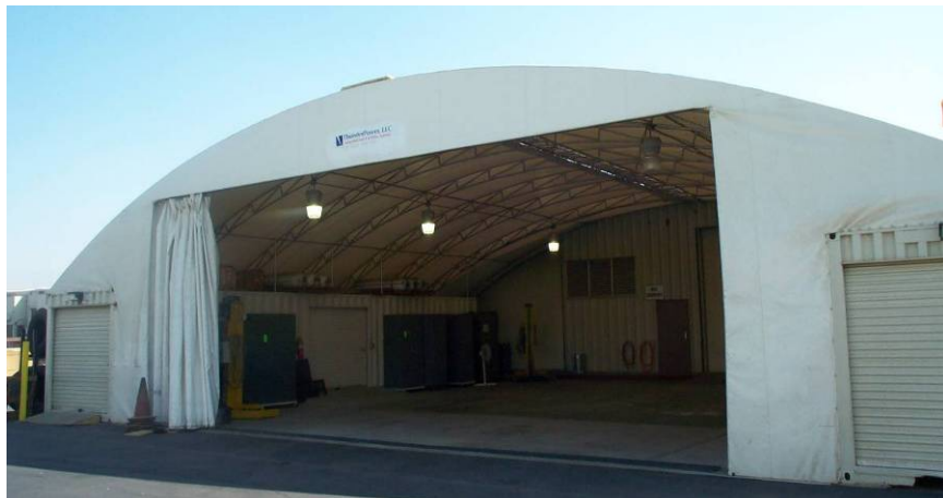
Figure C-11. Hydrogen maintenance building
