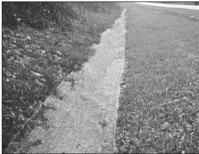
Figure 1.10. Installed Open Weave Textile Channel Lining
