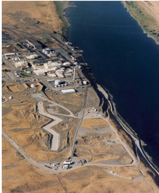
A liquid waste disposal trench (the Z-shaped trench) near Hanford's N reactor.
