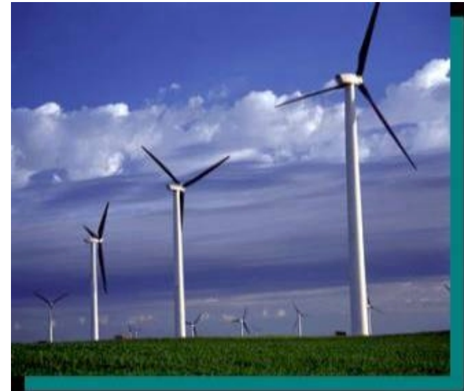
NSP 107 MW Lake Benton wind farm 4 cents/kWh (unsubsidized)
