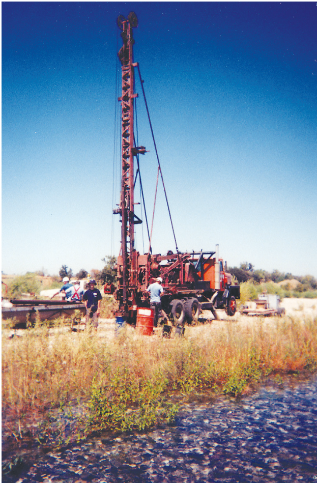
Figure 7. Photo of churn drill at site DPD-2, Daguerre Point Dam, California.
