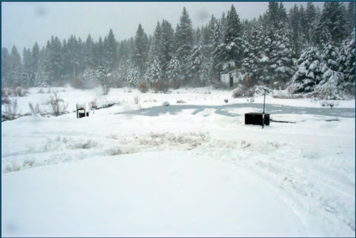
Cattleman's detention basin looking northwest. Photograph by James L. Wood.
