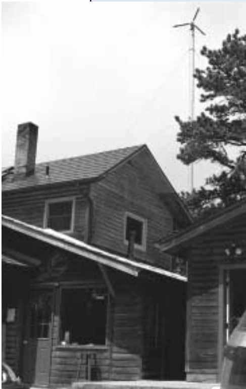
Jim Green, NREL / P1A12796
