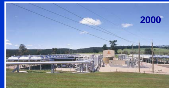
60 MW Mokai Combined Geo Power Plant, New Zealand
