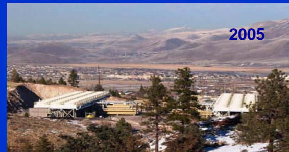
20 MW Burdette Binary Geothermal Power Plant, Nevada
