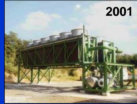
250 kW Geothermal Power Unit at Rogner Hotel & Spa, Bad Blumau, Austria
