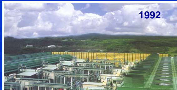
30 MW Puna Combined Cycle Geothermal Power Plant, Hawaii
