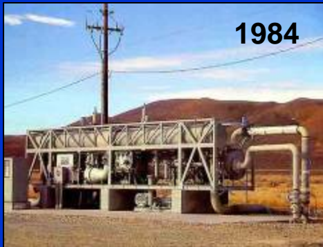
800 kW Wabuska Geothermal Power Unit, Nevada.
