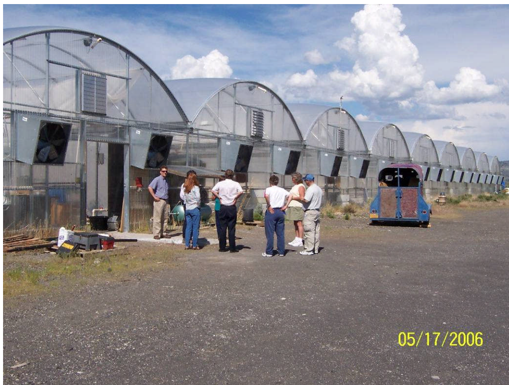
Attendees at newly restored geothermal greenhouse operation, Burns Oregon.
