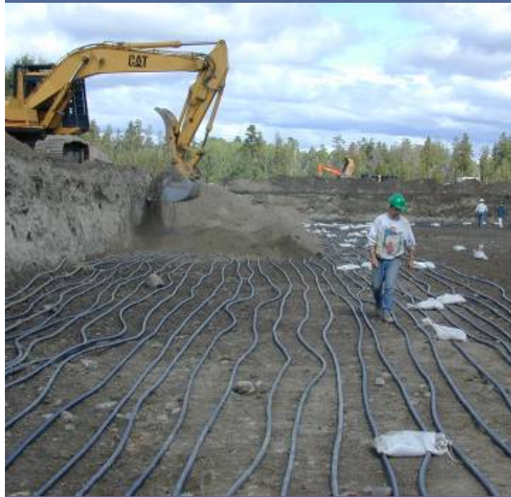
Excavation for a horizontal ground heat exchanger
