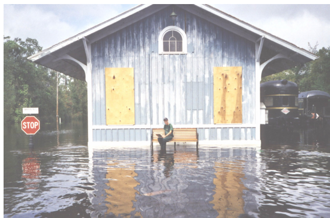
Flooding along the Waccamaw River due to Hurricane Floyd at railway station on S.C. Highway 905. Photo by Andy Caldwell on September 29, 1999.
