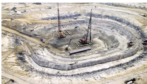
1964: Construction on A-2 Test Stand begins
