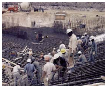
1964: Workers lay A-2 Test Stand base
