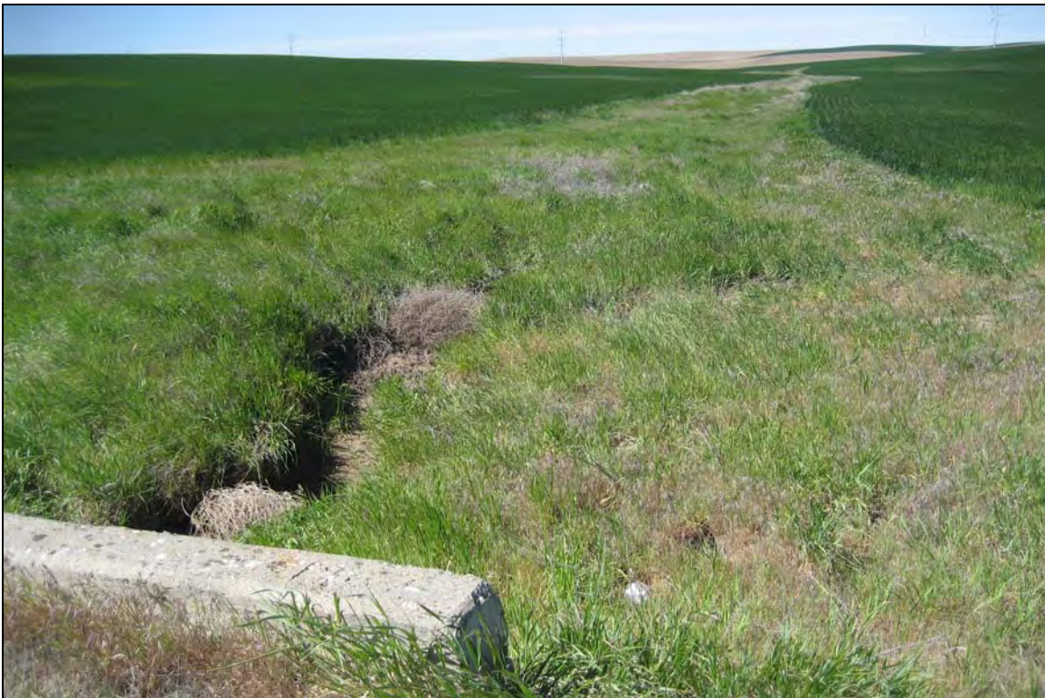
Photo Plate 6 View west, upstream, at stream crossing I, tributary to Biglow Canyon, upstream of stream crossing H.
