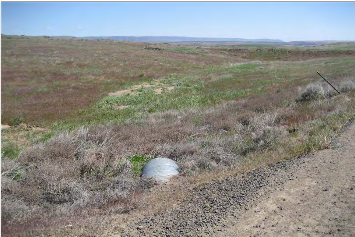
Photo Plate 8 View northeast, downstream, at crossing J, ESRI- mapped tributary to Biglow Canyon. Note earthen dam blocking drainage.
