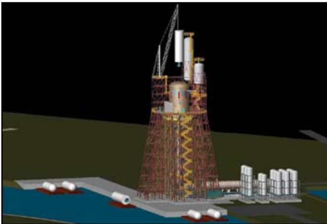
Artist concept of the A-3 Test Stand for testing the J-2X engines that will carry humans back to the moon.
