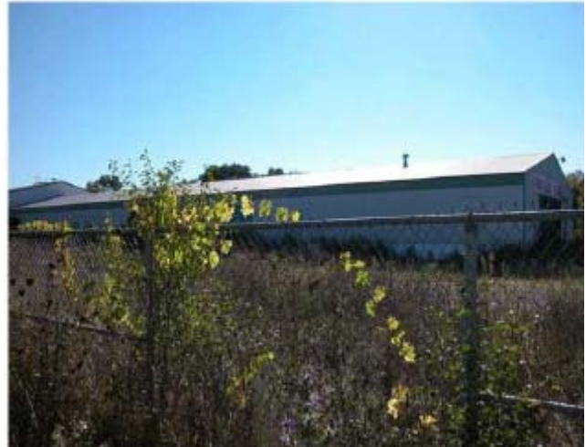
Central section, north facing side of the former processing building.
