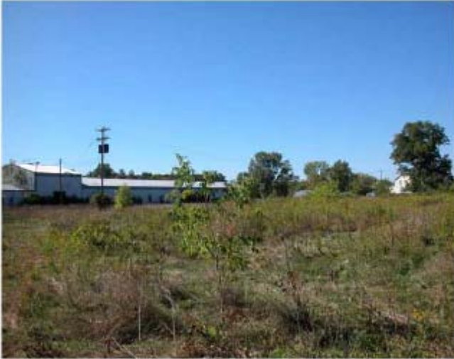
North facing side of former processing building.
