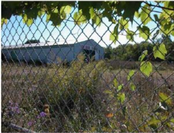
West end, north facing side of former Zonolite Co./W.R. Grace vermiculite processing building.
