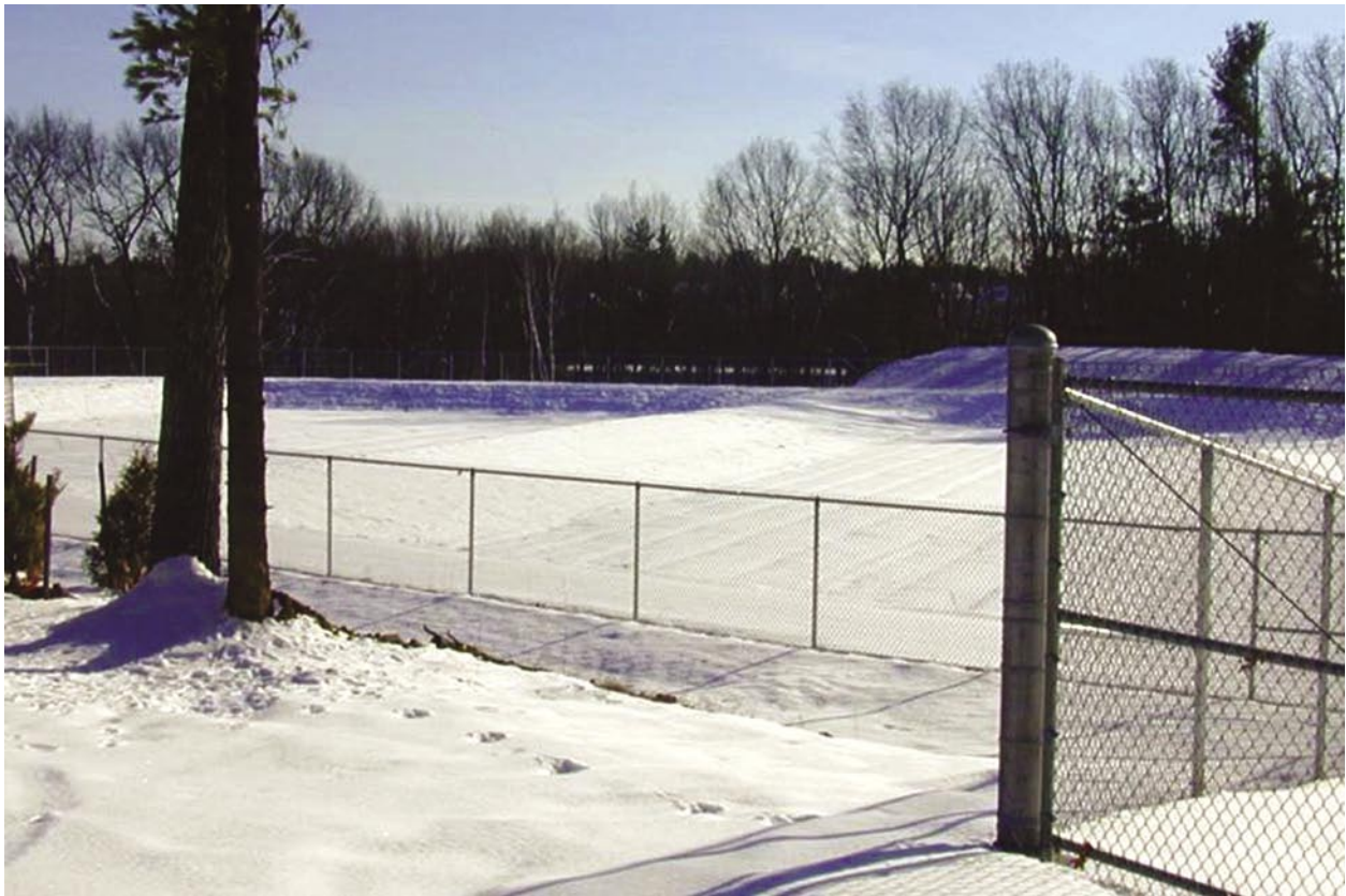
Figure 4. Sewage-infiltration beds at a new (2002) treatment plant in Acton, Massachusetts, permitted for a disposal rate of 0.25 million gallons per day.
