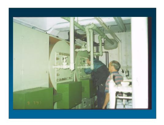
• Chlorine is the most commonly used disinfectant, but other oxidants are sometimes used and often have advantages over chlorine. The above photo shows ozone generators at a plant in the midwest. These particular ozonators have been in use since 1948, and are in especially good condition for their age. They are effective in removing tastes and odors as well as inactivating mircoorganisms.
