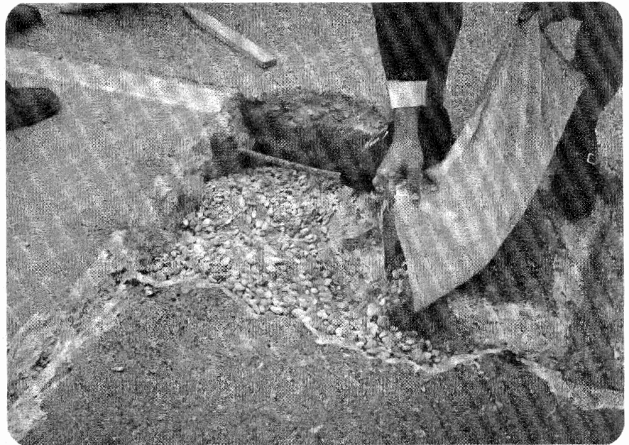
Figure 39. Placing coarse aggregate in the hole.
