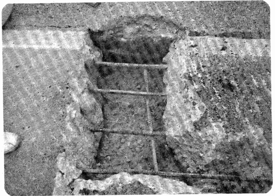
Figure 38. Hole prepared for polymer patch.
