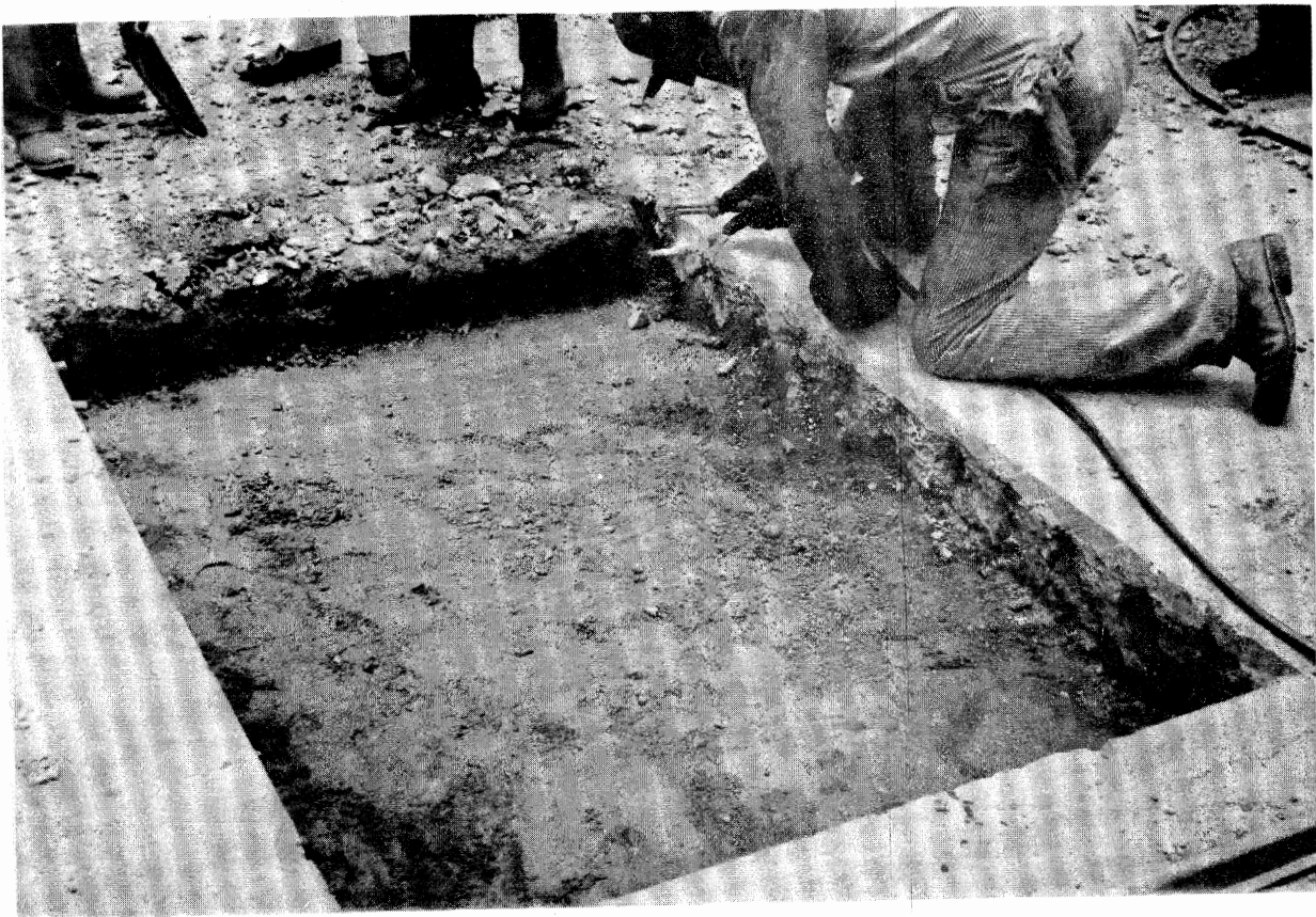
Figure 30. Preparing hole for precast patch.
