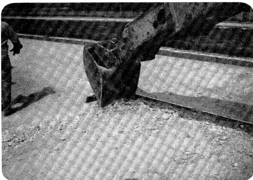
Figure 9. Preparing to lift out the slab in one piece.
