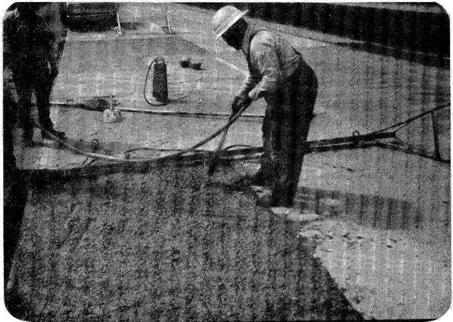
Figure 27. Vibrating the concrete.
