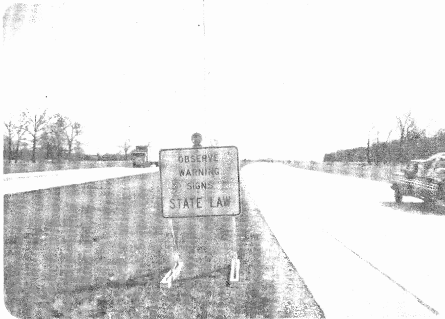
Figure 1. Advance warning sign (on both sides of the road).
