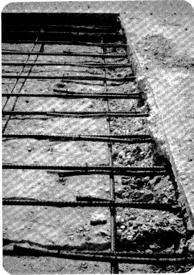
Figure 19. Typical tied steel splice.
