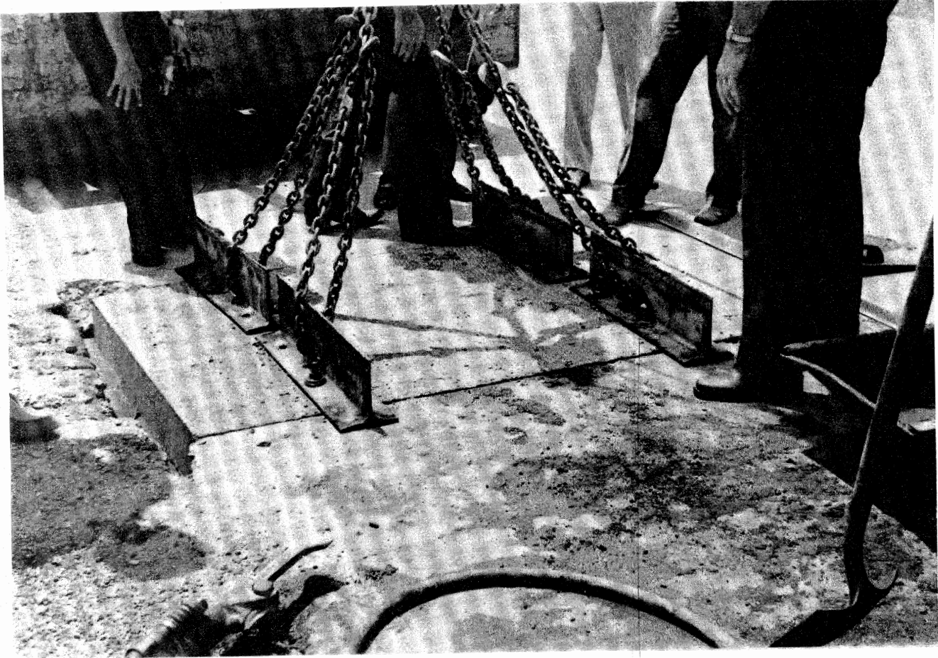
Figure 35. The slab in place.
