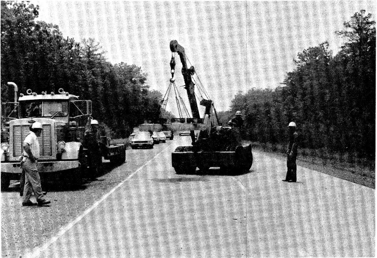
Figure 33. Taking the precast slab from truck to the hole.
