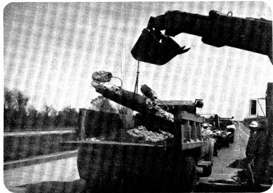
Figure 13. Loading the slab for disposal.
