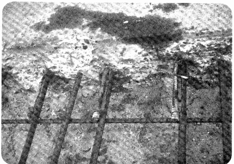
Figure 18. Typical welded steel splice.
