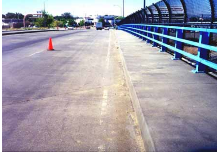
Figure 56. Lomas Boulevard westbound structure over I-40 (Albuquerque, NM).
