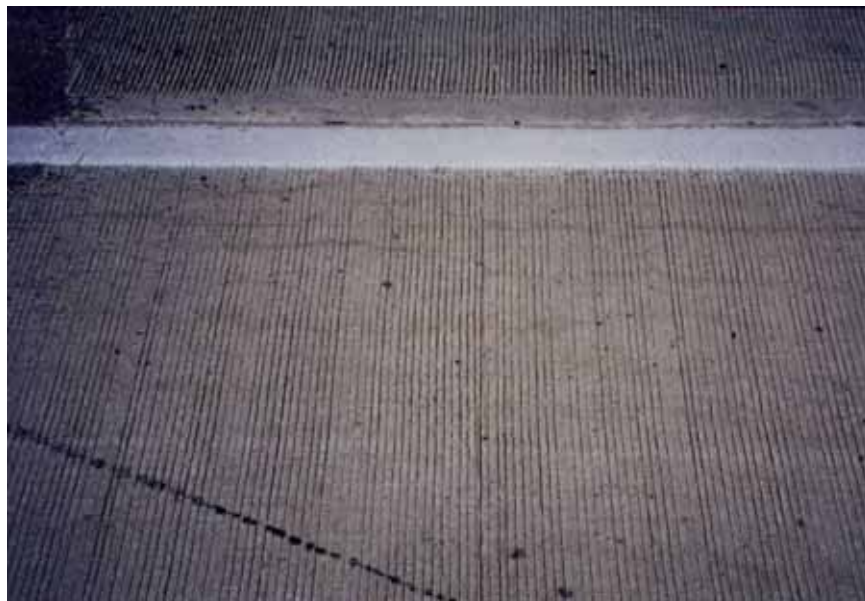
(i) Control section 5 (C5)
