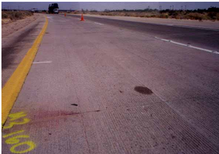
Figure 37. Photograph showing part of Boron, CA, test site, M3, Station 160.
