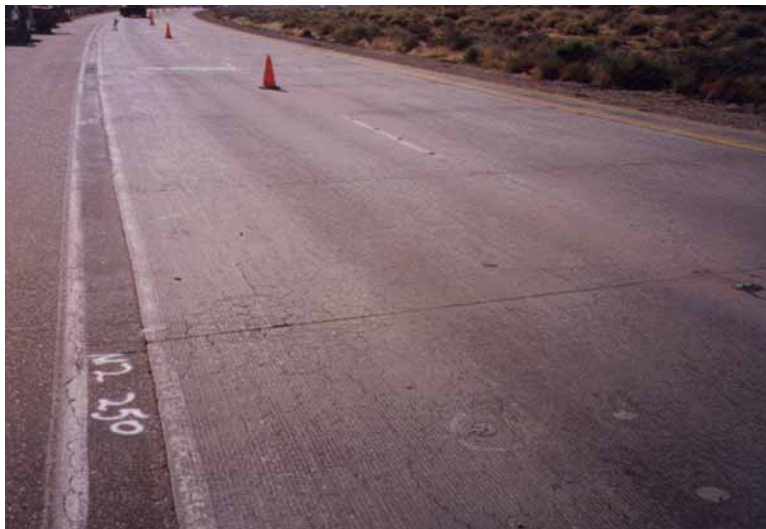
Figure 36. Photograph showing part of Boron, CA, test site, M2, Station 250.
