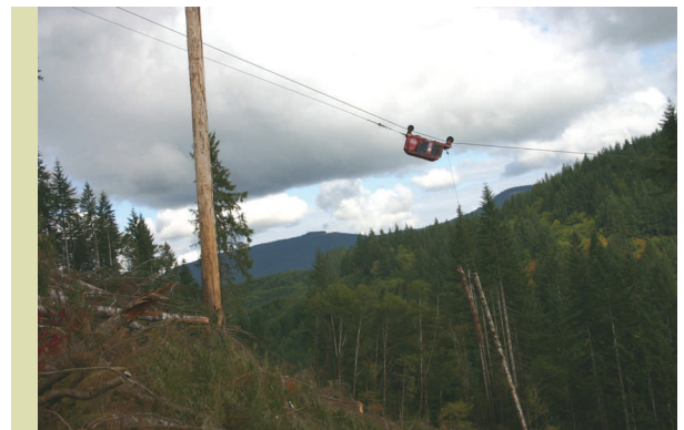
Logs preparing to be yarded for stream structure placement.
