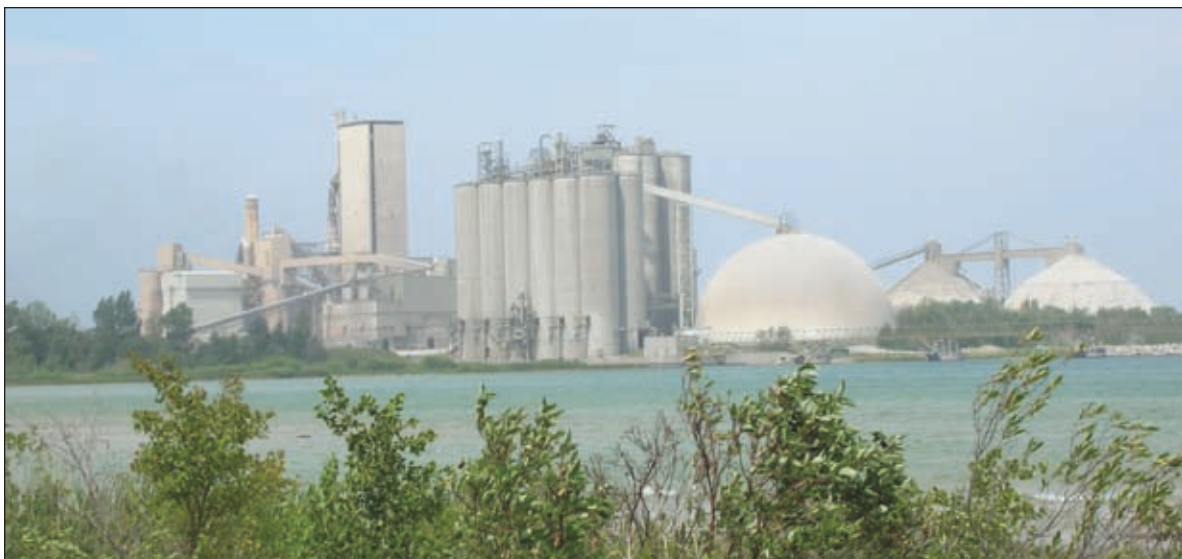
▲ Figure 8-9. Cement production and emissions. In addition to the emissions from energy consumption, a cement factory has direct process emissions of CO 2 that result from its conversion of limestone. Mitigation of process emissions of CO 2 and other greenhouse gases must also be considered in an economically efficient policy.
