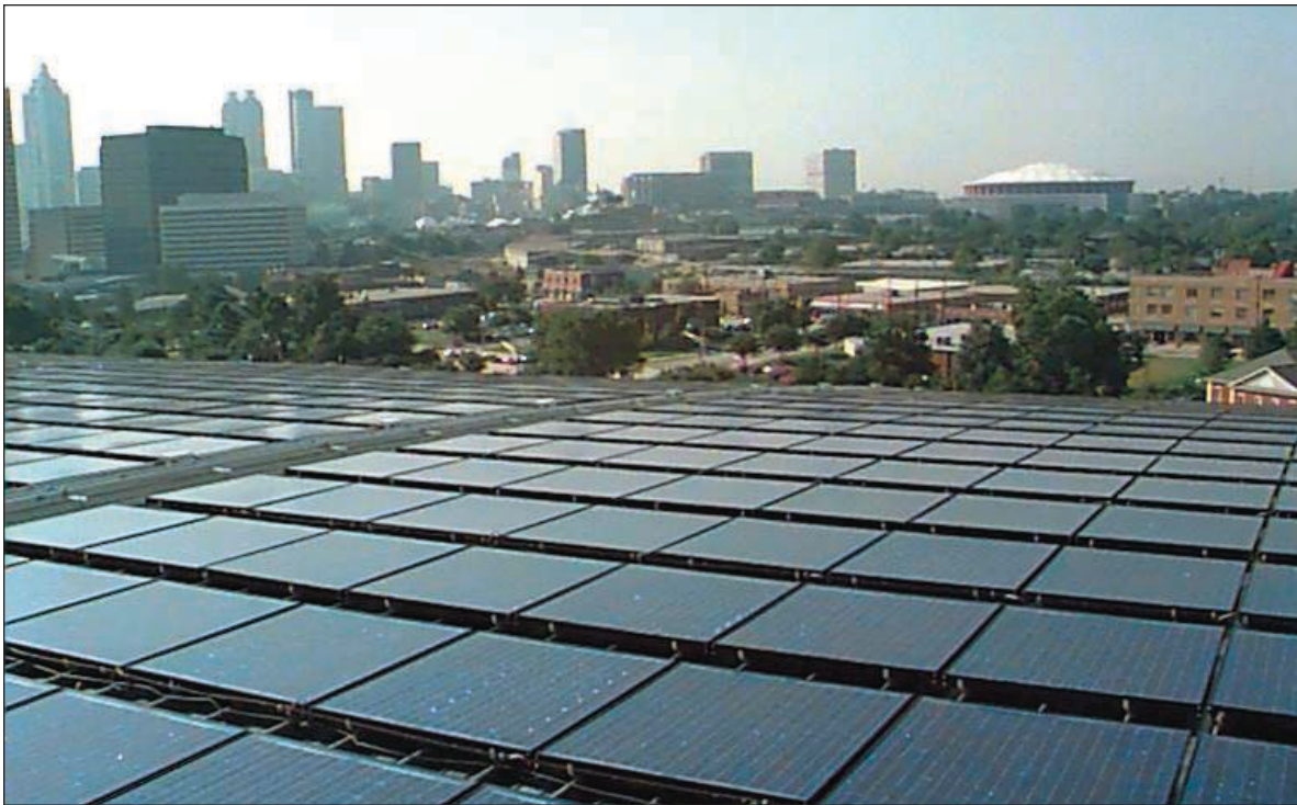
▲ Figure 7-4. An array of solar photovoltaic (PV) panels. PV is the most versatile solar technology. It can be deployed in any location, with output roughly proportional to the amount of sunlight.
