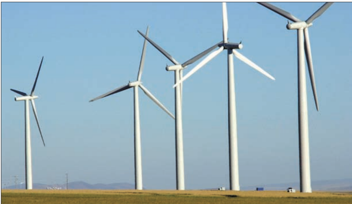
▲ Figure 7-2. An Array of Wind Turbines. Typical new wind turbine size is on the order of 1.5-2.5 megawatts (MW). Turbines are sited in wind farms to build economies of scale for transmitting electricity to load centers.
