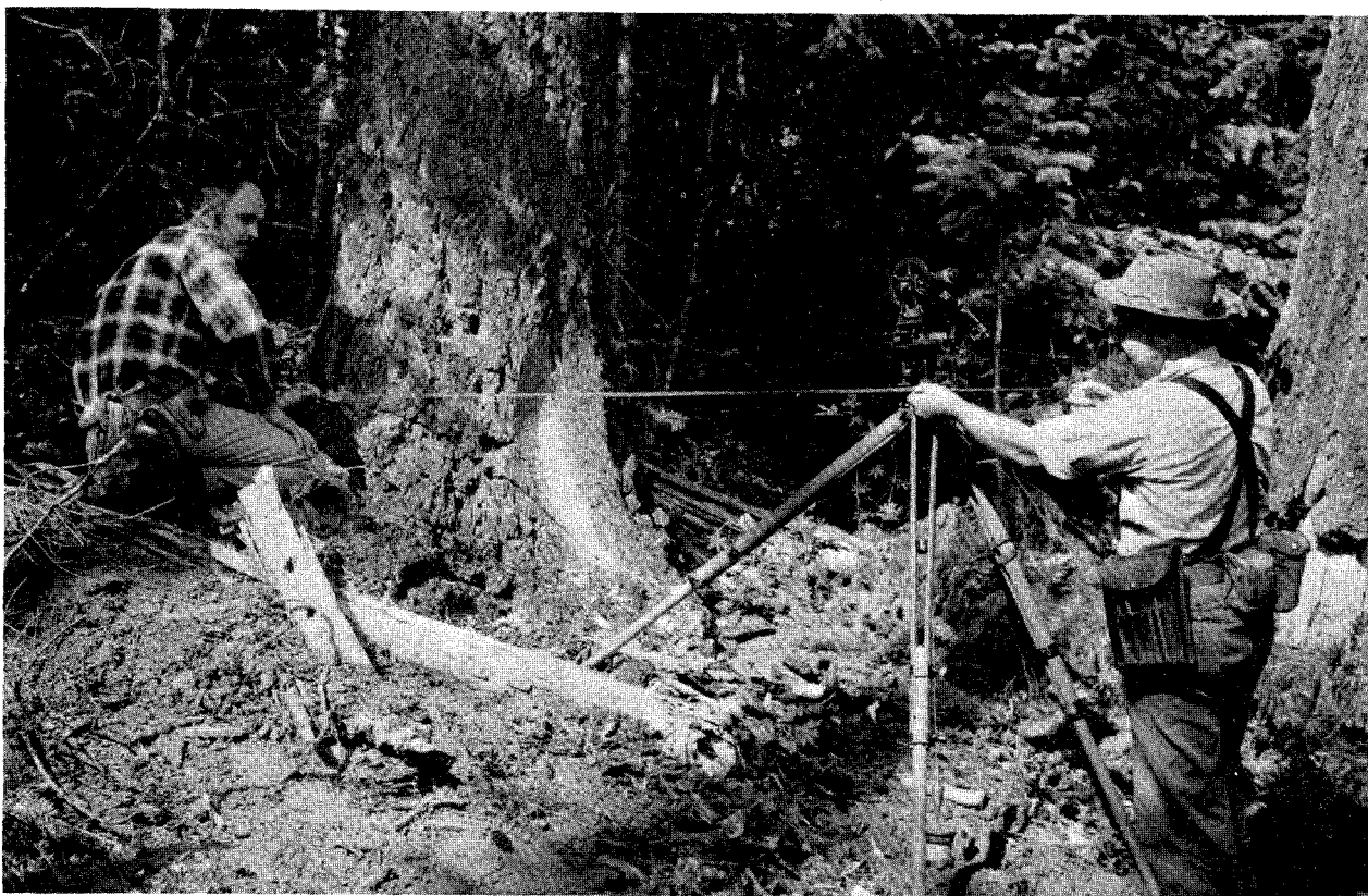
Marking a bearing tree.
