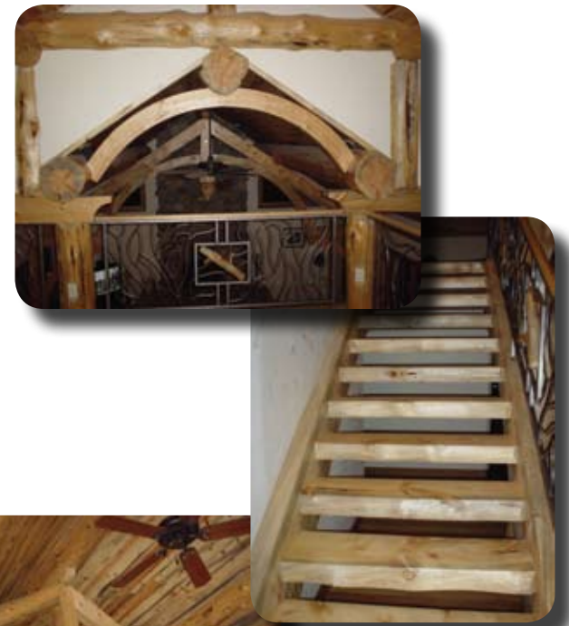
Examples of blue stain wood used in home construction
