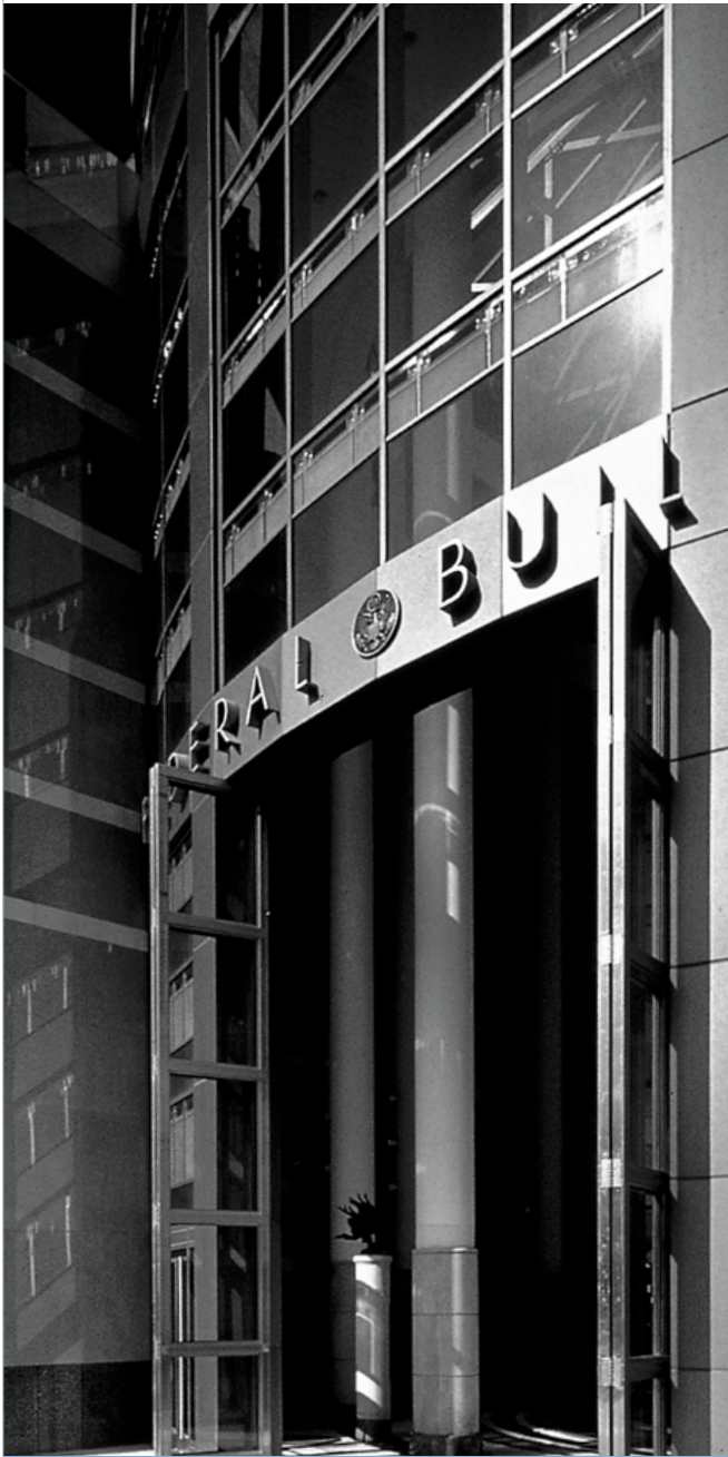
Oakland Federal Building, Oakland, CA.
