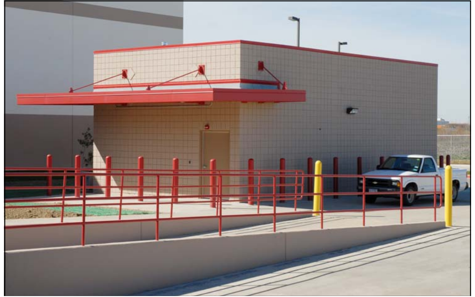
NARA-SW Region Electronic Records Storage Vault. (Photo by Steve Ourada)
