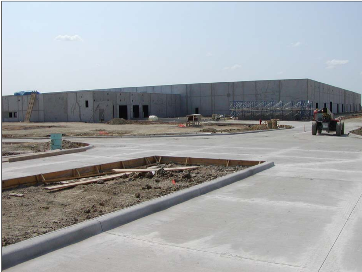
New Regional Records Center Construction Site - August 2006
