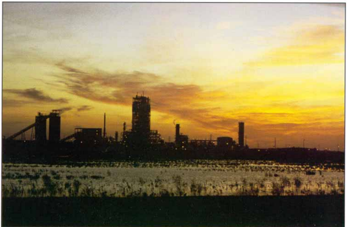
Dawn arrives over the reclaimed wetlands surrounding the Tampa Electric Integrated Gasification Combined-Cycle Project
