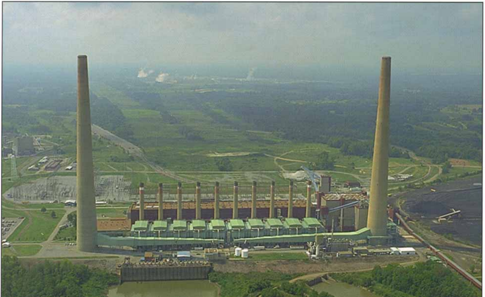
The host site for the GSA demonstration is TVA's Shawnee Fossil Power Plant near Paducah, Kentucky.
