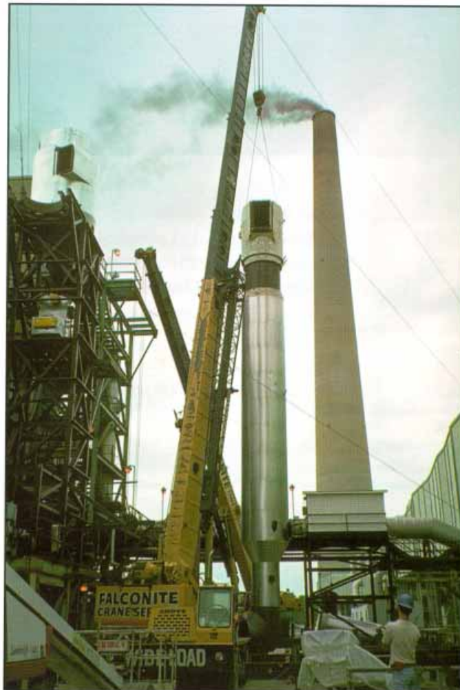
The insulated GSA reactor is being lifted into place during construction.
