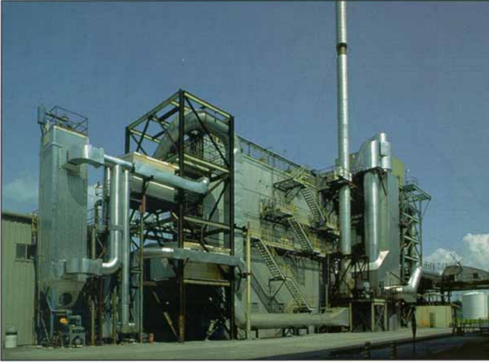
The Clean Coal GSA Demonstration Site at Paducah, Kentucky.
