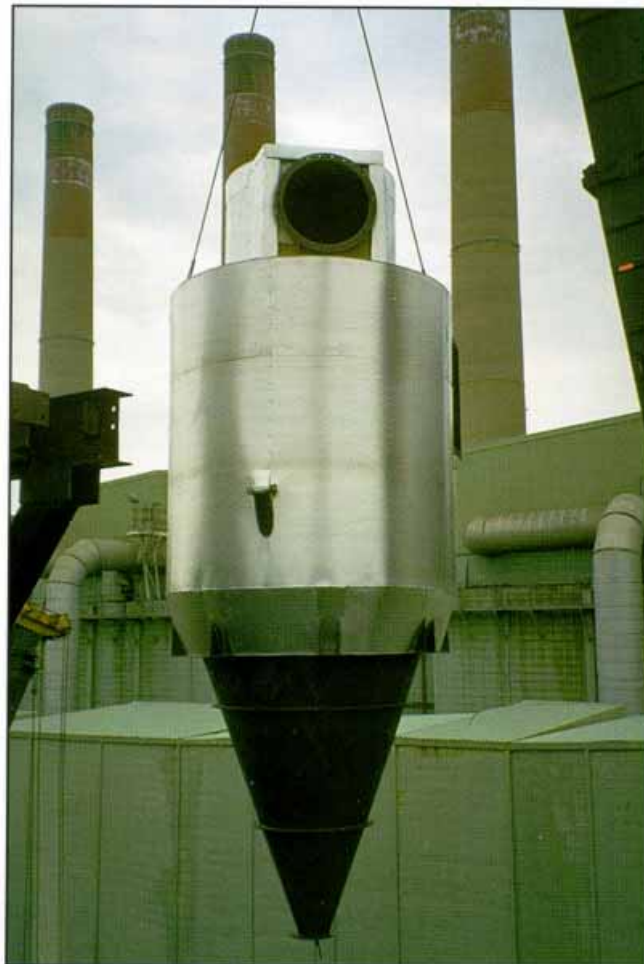
Insulated cyclone separator being elevated for placement into the system.
