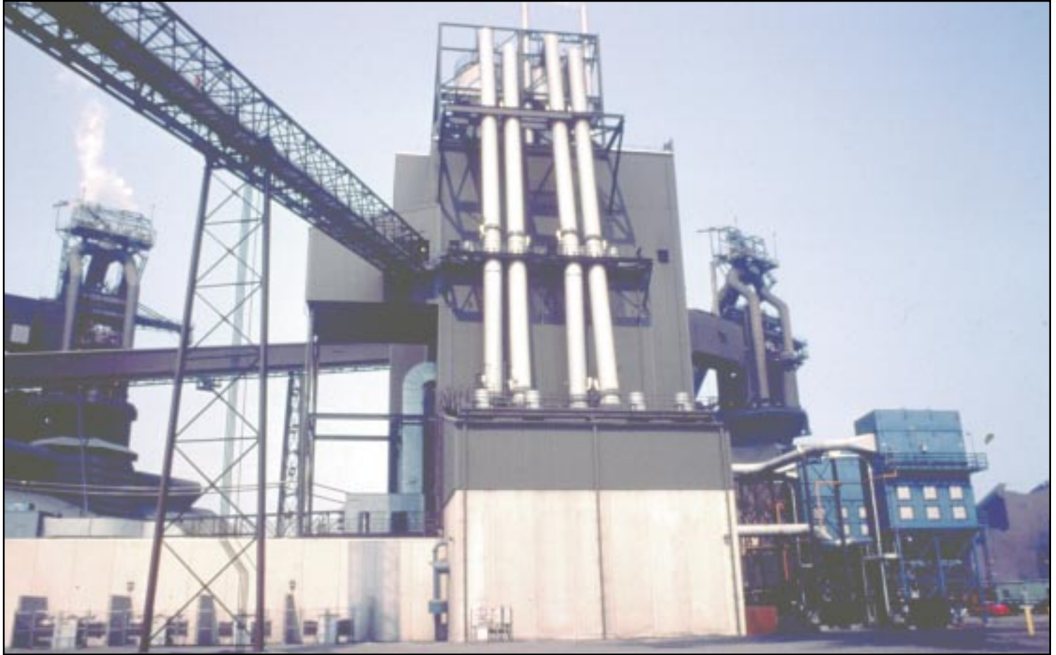
Granular coal preparation building with blast furnaces in background
