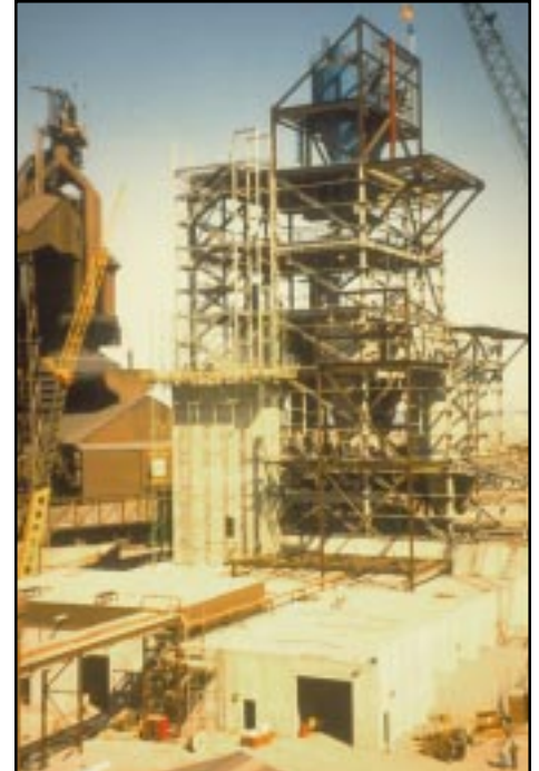
BFGCI demonstration facility under construction
