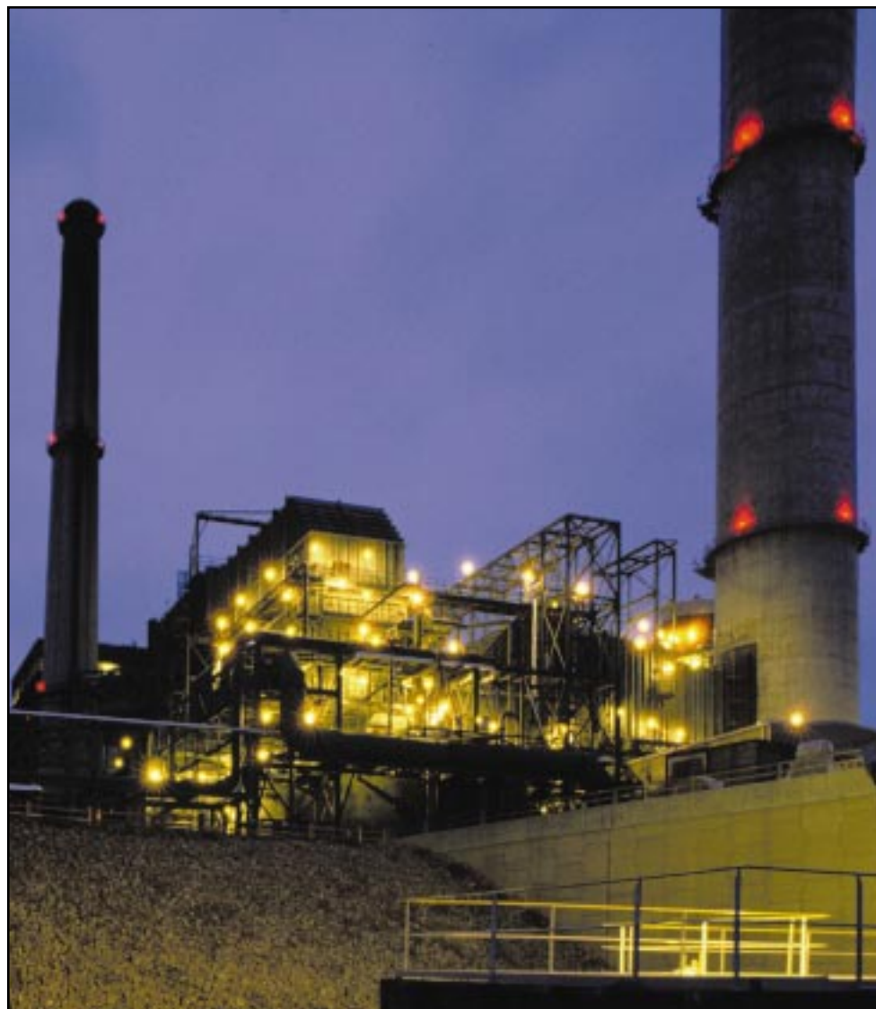
Night view of Bailly Generation Station.
