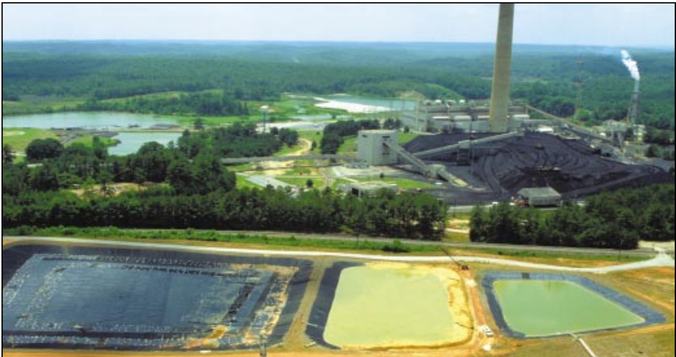
Aerial view of Yates Electric Station.
