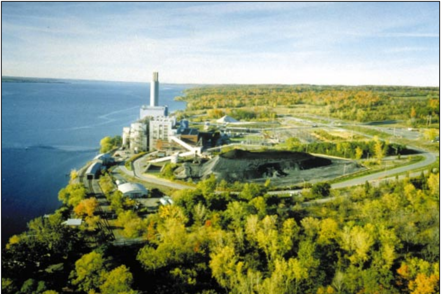
Aerial view of Milliken Station.
