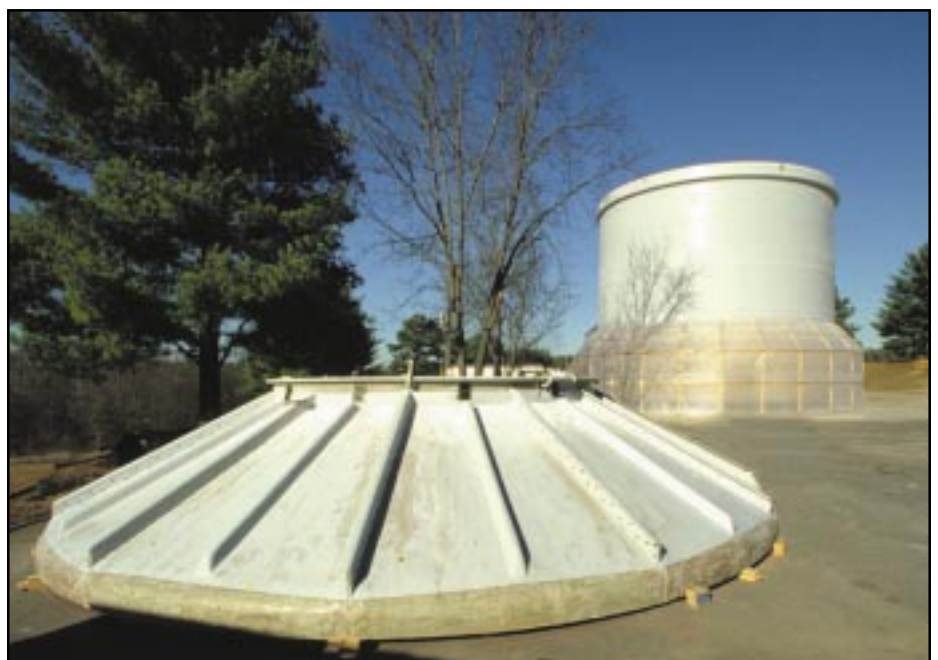
Yates CT-121 scrubber in the early stages of fabrication.
