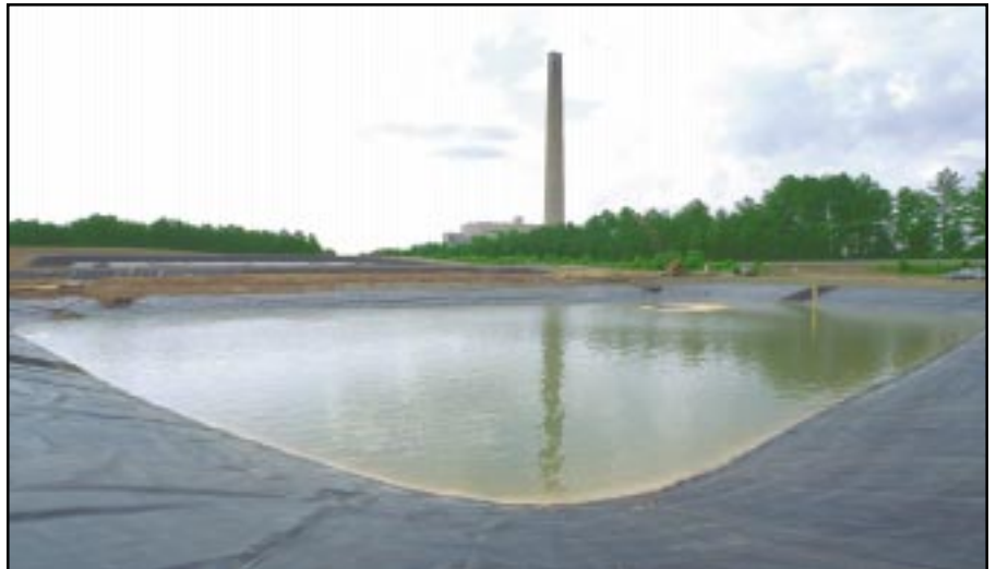
Gypsum stack impoundment at CT-121 Demonstration Unit.
