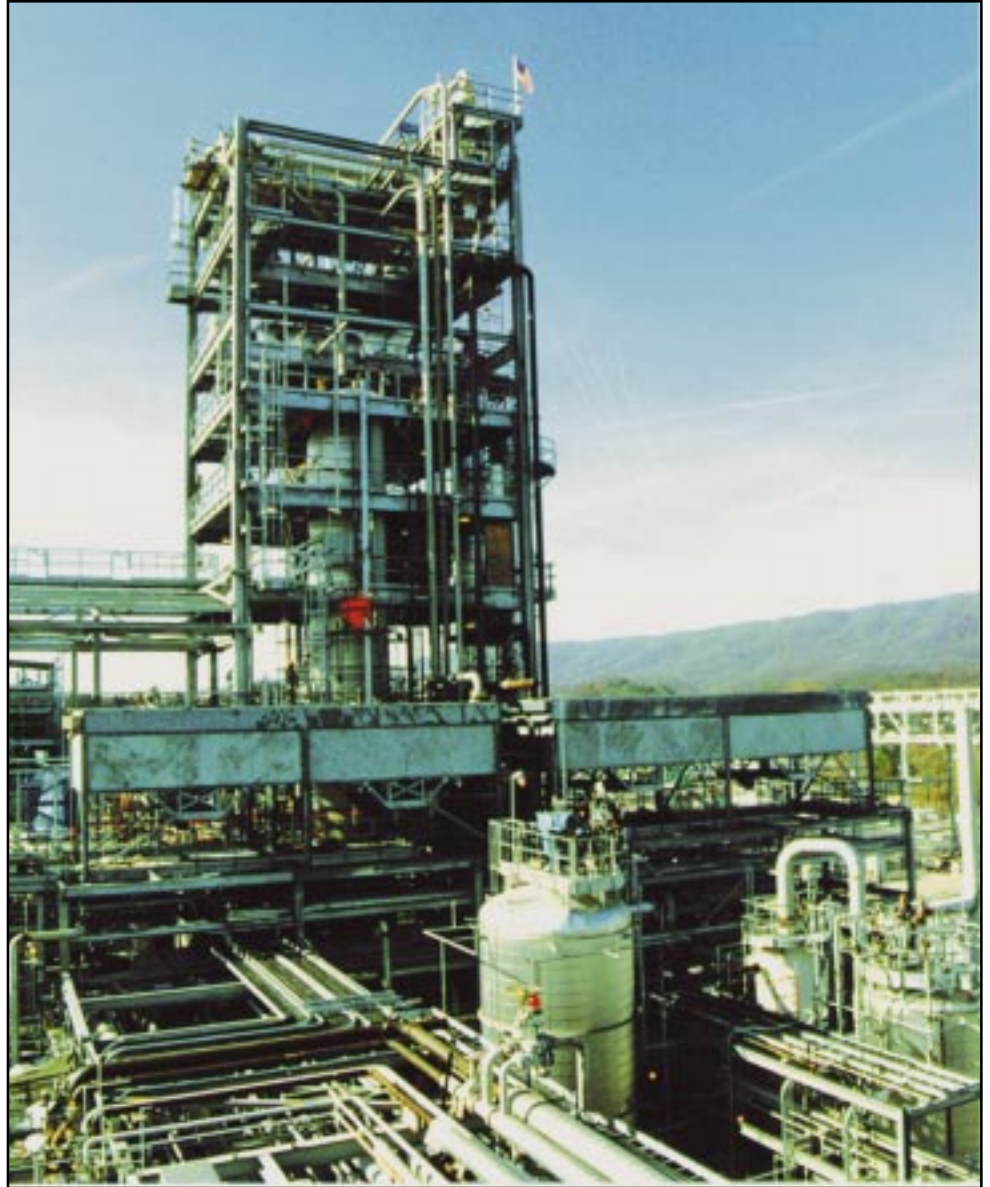
LPMEOH™ Demonstration Unit.
