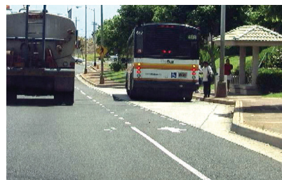
Bike lane on Farrington Highway, Kapolei, Oahu.
