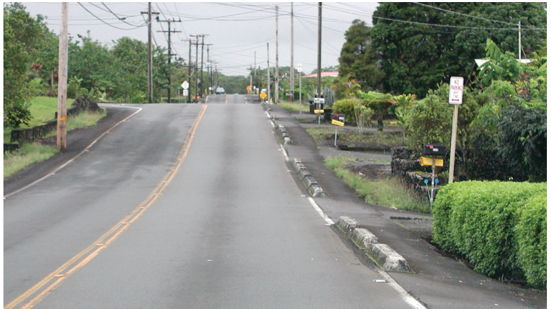
Asphalt berms separate motorized and non-motorized travel ways on Puainako Street, Hilo, Hawaii.
