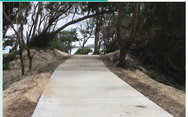
Bike and pedestrian path, under construction, Lydgate Park, Kauai.
