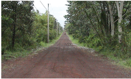
This section of the proposed Railroad Avenue Bikeway, which passes through the Hawaiian Paradise Park subdivision, is composed of packed crushed cinder and currently used for local vehicular circulation. Puna, Hawaii.
