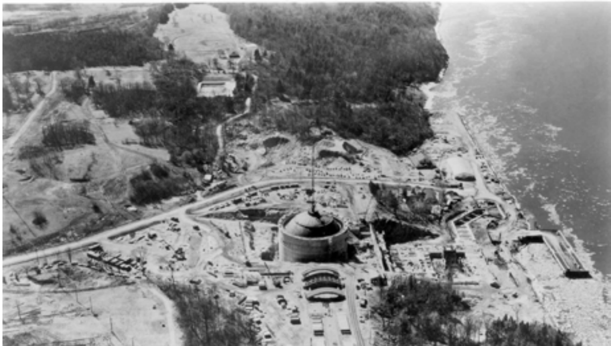
Construction of Indian Point 1
