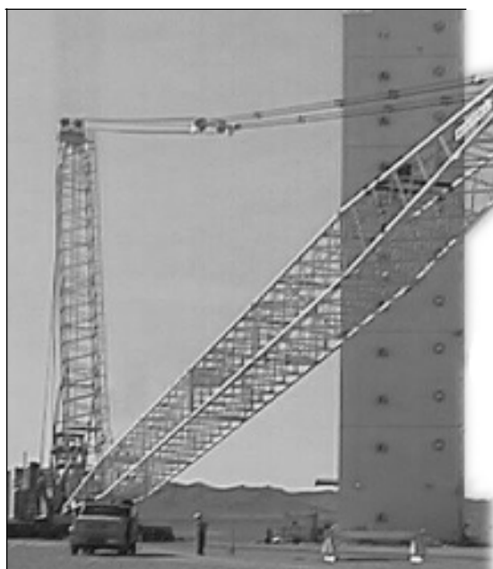
LLNL's big crane moves to Chestnut Ridge.
