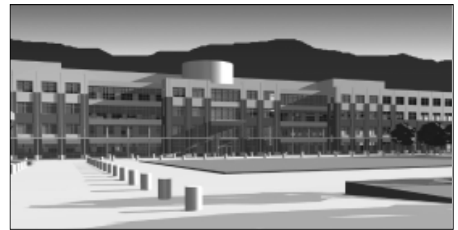
Artist's concept of the privately funded facilities, a key element of ORNL's modernization
