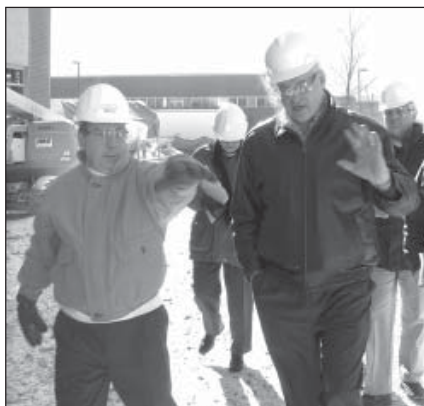
On a chilly day, Bill Madia (left) takes Battelle CEO Carl Kohrt on a tour of east campus construction.
