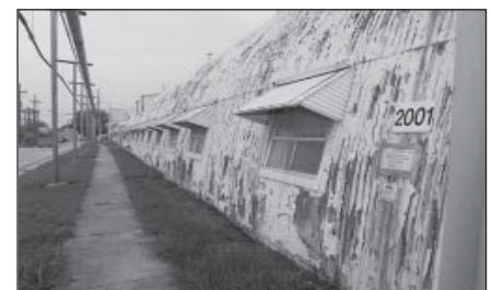
Building 2001, the “Winter Palace”
