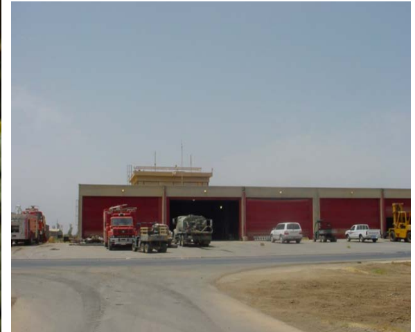
New Fire Station – Observation
