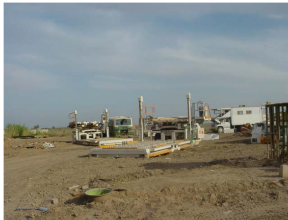
Wrecked GSE – Adjacent GSE Workshop
