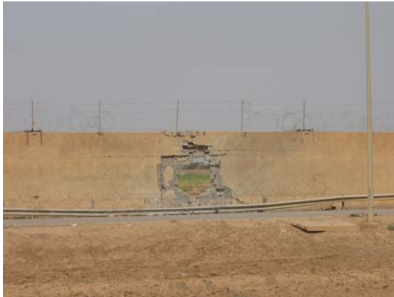
Perimeter Fence – Breach
