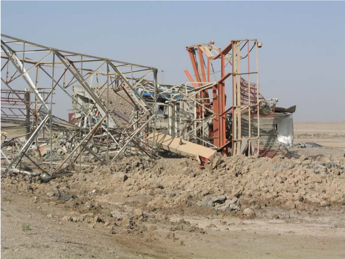
Destroyed SSR facility
