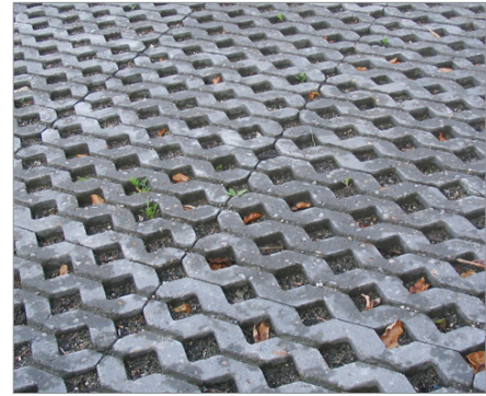
Utilize pervious paving to allow stormwater to infiltrate on site, rather than flood property or create site run-off.
