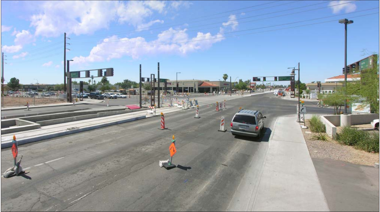
Figure 28: Existing conditions along Apache Boulevard looking west towards McClintock Drive
