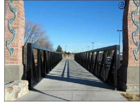
A grade-separated pedestrian crossing
