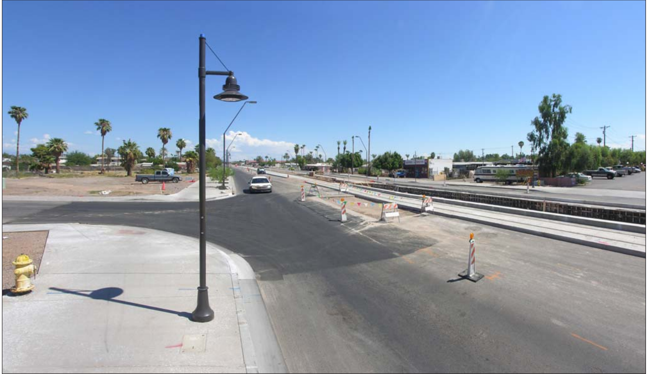
Figure 39: Existing conditions along Apache Boulevard looking east toward Smith Road
