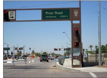
LRT construction on Apache near Price Road
