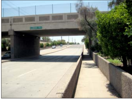
McClintock Drive railroad underpass
