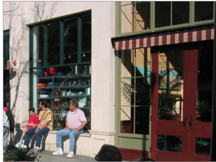
Articulation in the form of an integrated seatwall and an attractive display increase and enhance the interaction between pedestrians.
