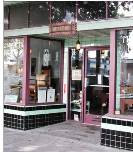
Figure 8: Recessed storefront entrances and small entry plazas for residential or office buildings allow greater mobility and expand the utility of narrow sidewalks.
