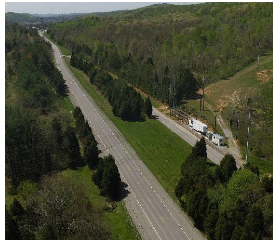
Fig. A.9. Aerial view of the PCAT Facility.
