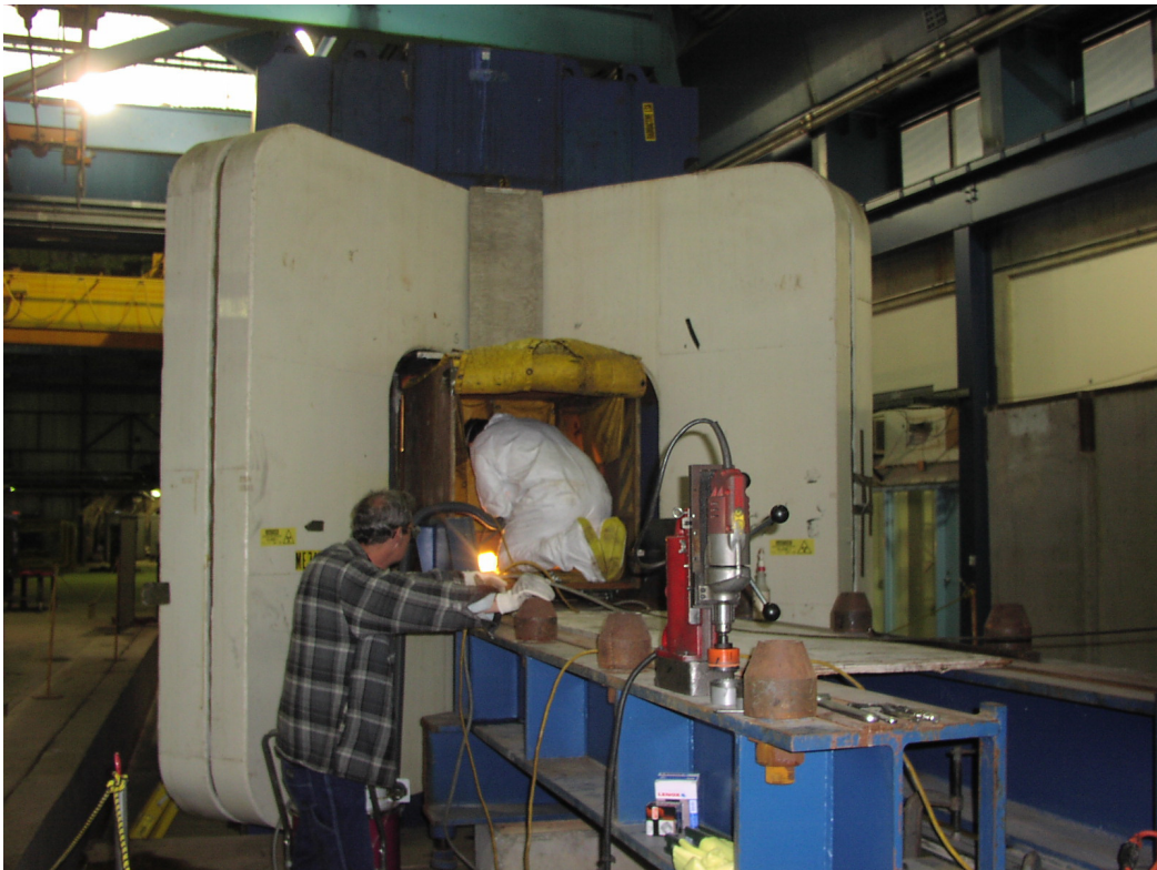
Worker Inside Shielding Fixture within SM12 Magnet Beam Cavity
