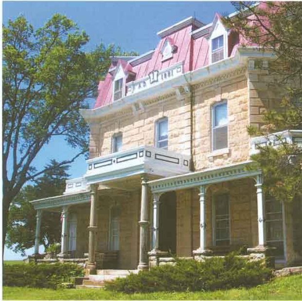
The Spring Hill Ranch house built with native Cottonwood limestone
